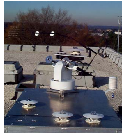
Figure 7 Roof Top Meteorological Station
