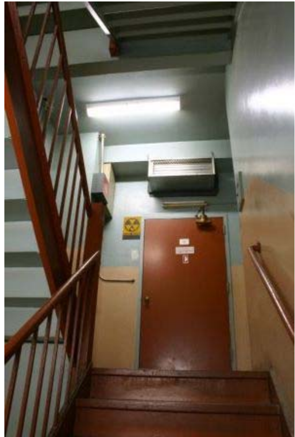
Figure 18: Staircase C landing, 34 th floor
