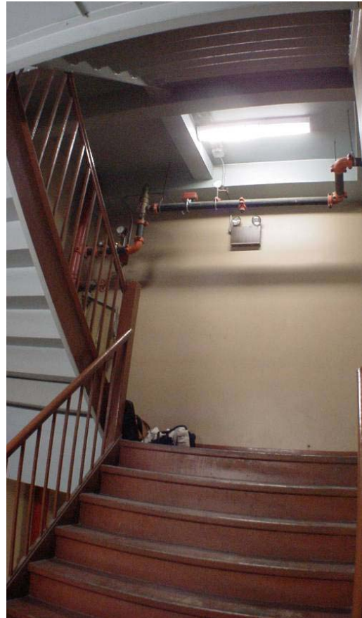
Figure 12: Staircase A, 11th floor landing
