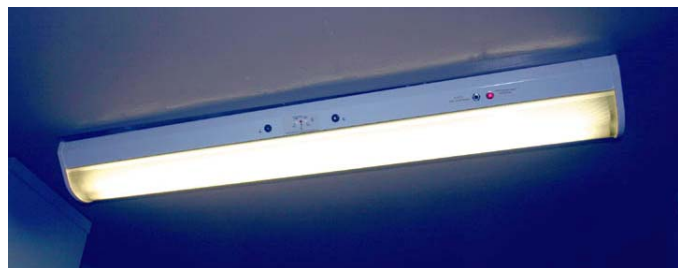
Figure 2: Occu-smart fixture (showing ultrasonic transducers)
