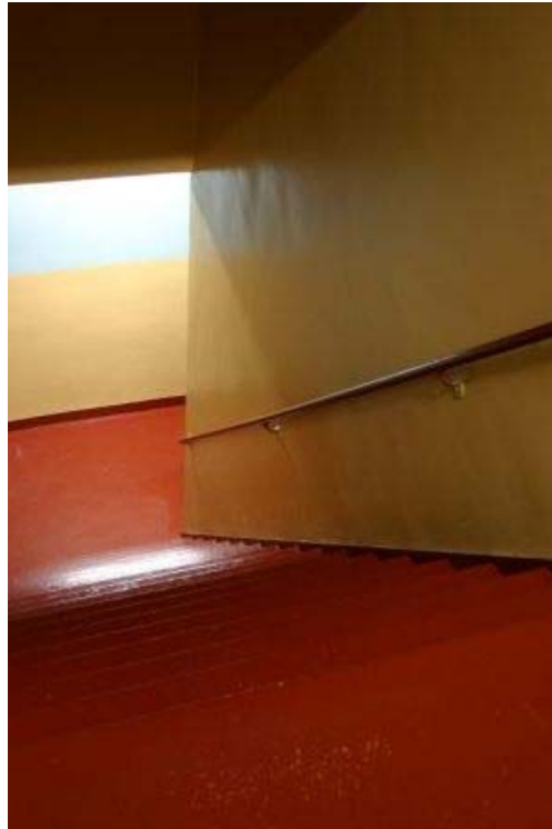
Figure 14: Staircase A (Straight Run), looking downward
