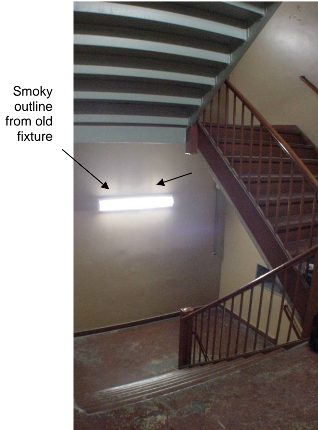
Figure 11: Staircase A, mid-landing between 10-11th floors
