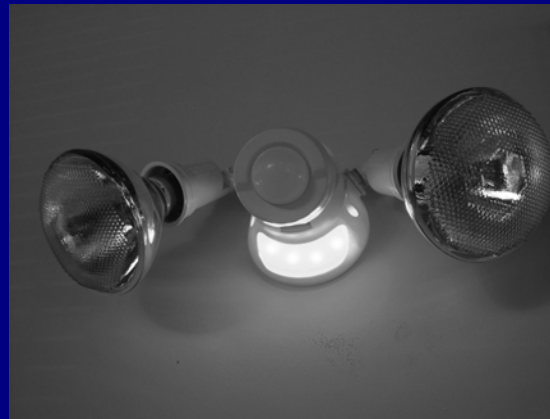
The 5-Watt LED array provides continuous illumination
