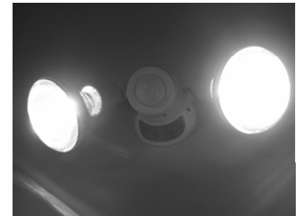
Motion sensor activates flood lamps
