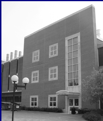
Field study site: Empire State Hall at Rensselaer Polytechnic Institute.
