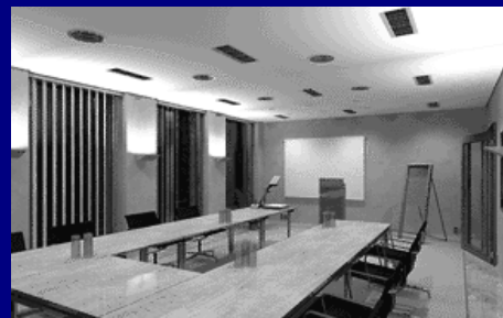
DALI allows for different preset "scenes" as shown in these photos.
