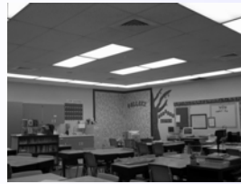
The pre-retrofit classroom system is shown on the left with lensed troffers. The new ICLS system is shown on the right.
