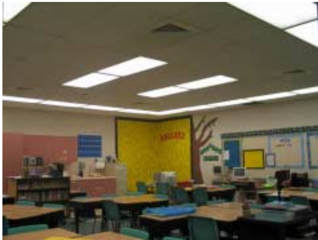
Energy Use Before 1.75 watts / sq foot
